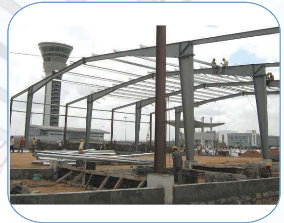
CIVIL WORK ON SITE
